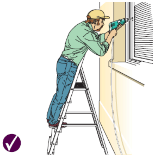
Figure 3a Correct - rungs facing work activity
